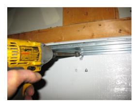
Slide the top of the opener bracket under the strut where you removed the screw earlier.
