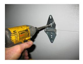
Remove the screws from the center of the top strut just above your original bracket.
