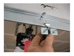
Unplug the garage door opener and remove the old bracket from the door. If the inside of the door is bent straighten the steel.
