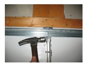
Secure the lower portion of the bracket **OVER** the hinge as shown, and secure with existing screws removed earlier.
