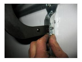
Secure the bottom of the opener arm to the opener bracket by sliding the pin through one of the holes in the bracket. Secure the pin with the pin keeper.
