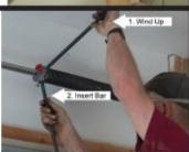
Stretch the springs the thickness of a coil and tighten the set screws.
