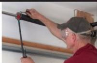
CAUTION! To prevent the door from knocking you off the ladder, carefully follow these procedures. 1. Remove the first vise grip from the track. If the door rises, remove tension from the springs until the door stays closed. 2. Remove the second vise grip from the shaft.
