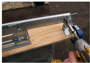
Check the track-to-jamb dimension and adjust the distance here so it is the same as your existing track-to-jamb dimension. This will be the same dimension you provided for ordering the high lift kit.
