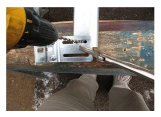
Bolt bracket to track. Lay down the high lift extension system on a flat surface (as shown) because both the bracket and the angle should be on the same plane, as they will both be attached to a door jamb.
