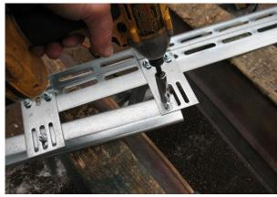
Assemble JB bracket with a #8 splice plate.
