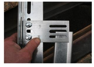
Drill two quarter-inch holes through the center slot onto the track.
