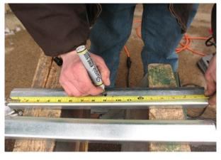
Drill hole where you marked center of track. Drill holes through tracks separately; do not attempt to drill through tracks while they are still paired together.
