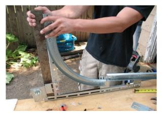
With the high lift track lined up with the square, measure from the horizontal track angle to the edge of the high lift angle. In this case, the distance is 2 7/8".
