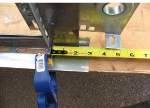
The plates now need to be adjusted for this distance. From each plate-angle junction, make a marking on the angle the same distance away (2 7/8") as the distance between the horizontal track angle and the edge of the high lift angle, measured in the previous step.
