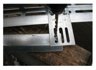
Secure plate onto track with track bolts coming up from underneath, and tighten with quarter inch flange nuts. Make sure track bolts are all the way out. An impact wrench is being used to tighten the nuts here, but a ratcheting wrench also works.
