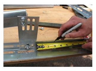
Remove nuts and bolts and slide plates to this marking.
