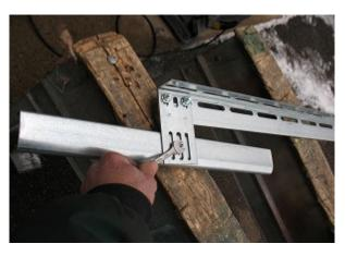
Position higher-numbered high lift plate so that the top edge of the track splits the center slot. Secure with 5/16" carriage bolts and flange nuts.
